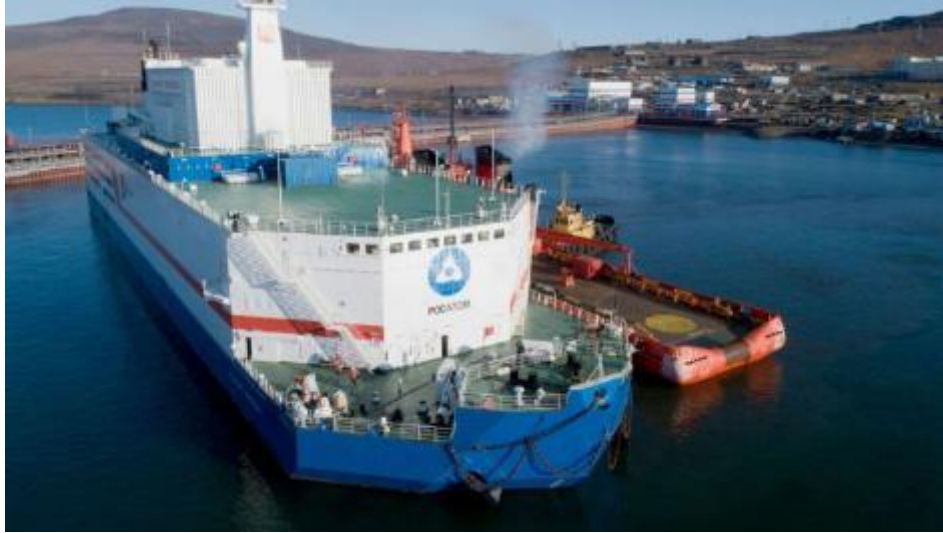
Figure 3 Akademik Lomonosov floating nuclear power plant
